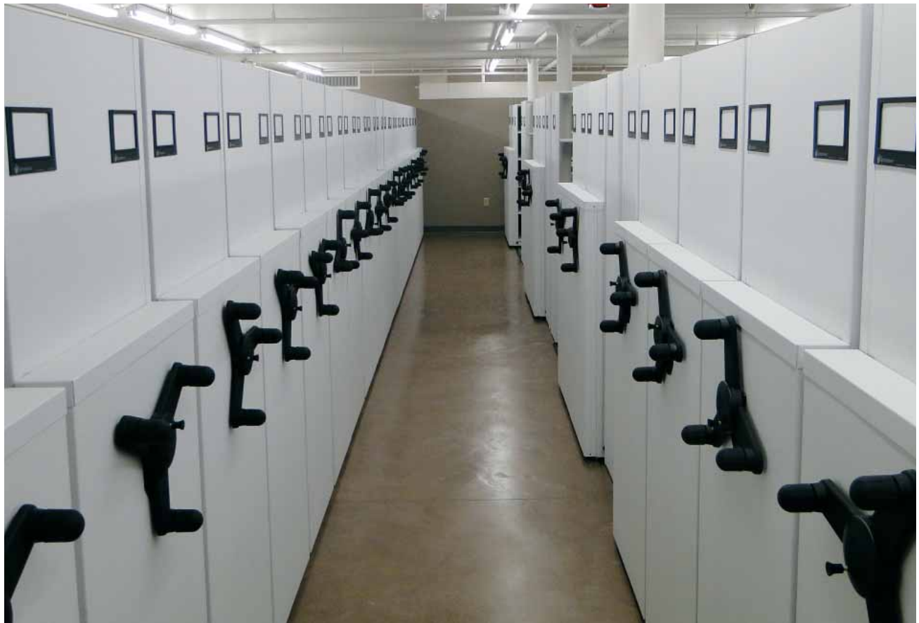
Recently installed lower level OSA repository.
